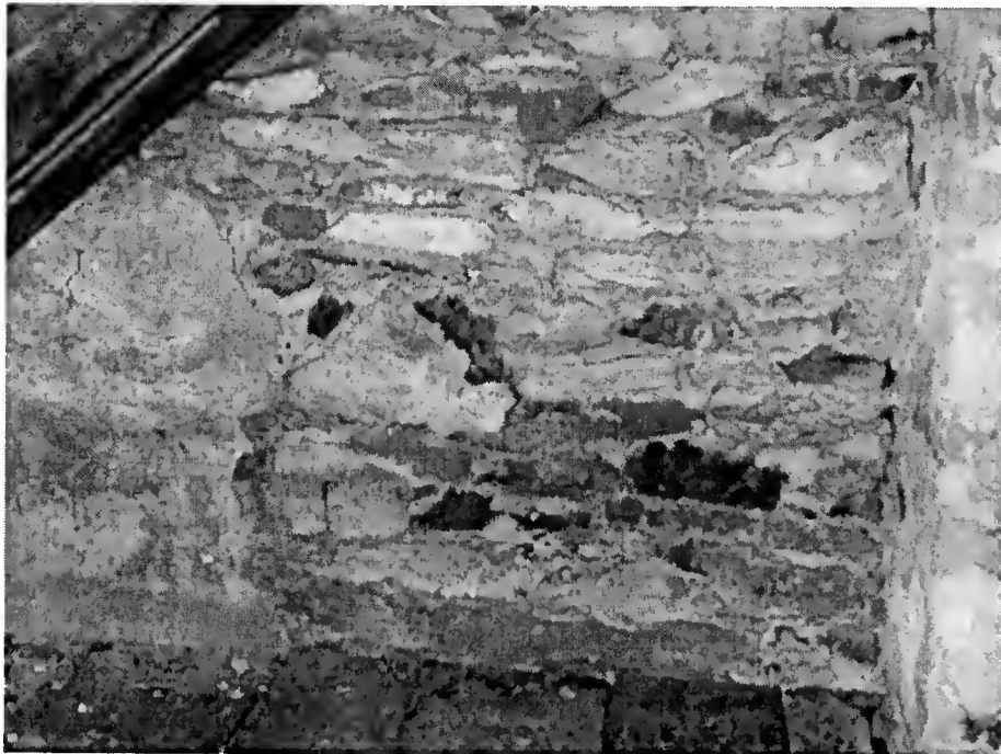
Figure 35 North Gable-End Wall in Attic of the Center Section of the Main House, 2002
